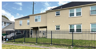
BLODGETT Project Cost: $420,000 Earning: $88,200/y Completion Time: 8 months
