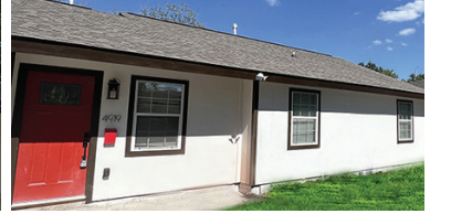
COSBY II Project Cost: $275,000 Earning: $52,560/y Completion Time: 7 months
