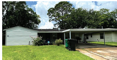
KELSO Project Cost: $203,000 Earning: $39,600/y Completion Time: 4 months
