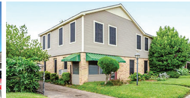
ISABELLA Project Cost: $390,000 Earning: $63,000/y Completion Time: 11 months
